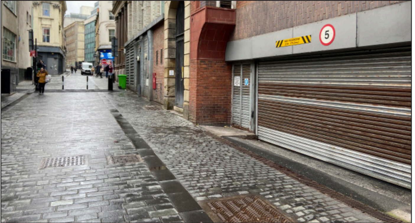
CAR PARK ENTRANCE ON HARRINGTON STREET
