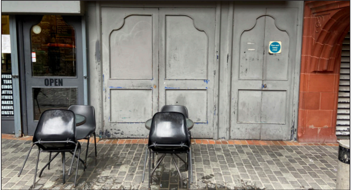
GOODS LIFT (DOUBLE GREY DOORS - HARRINGTON STREET)
